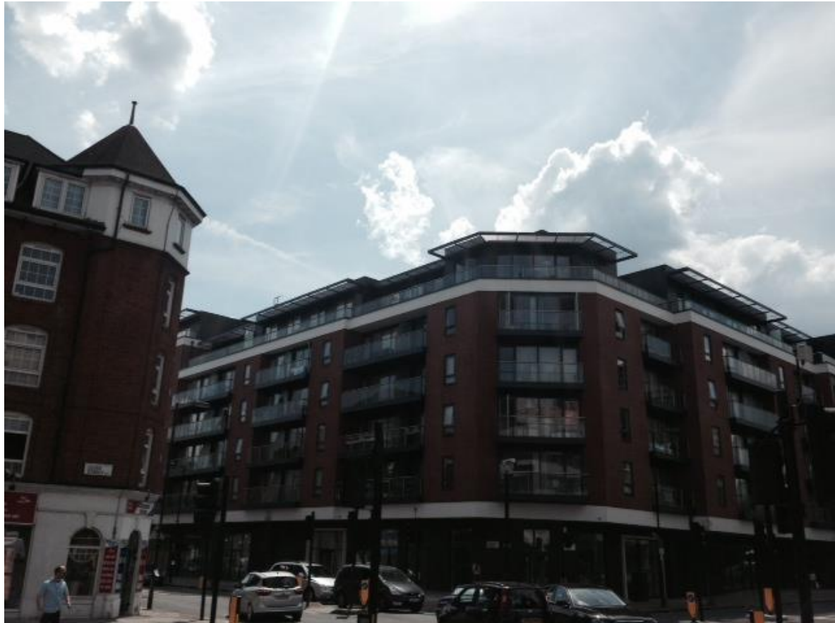
Image 2: View from the corner of Central Street and Lever Street
